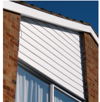
3. Fit first plank at base
